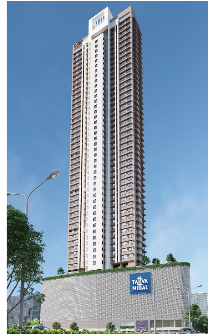
MITTAL SKYE | DADAR | TMGL STATUS: UNDER CONSTRUCTION
