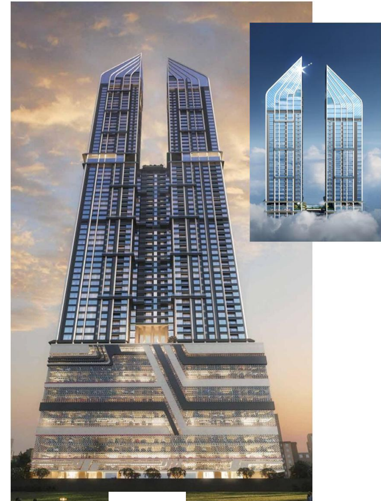
SHREEPATI SKIES- ADADHYA AVAAN | G+80 | GIRGAUM STATUS: UNDER CONSTRUCTION
