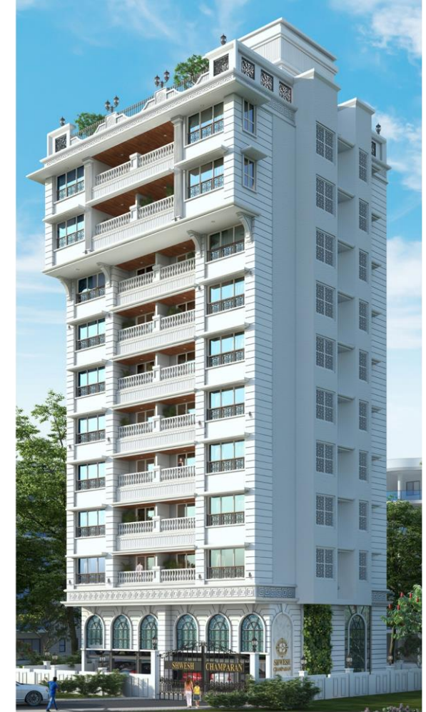
SHWESH CHAMPARAN | MATUNGA STATUS: UNDER CONSTRUCTION BNSA + SC
