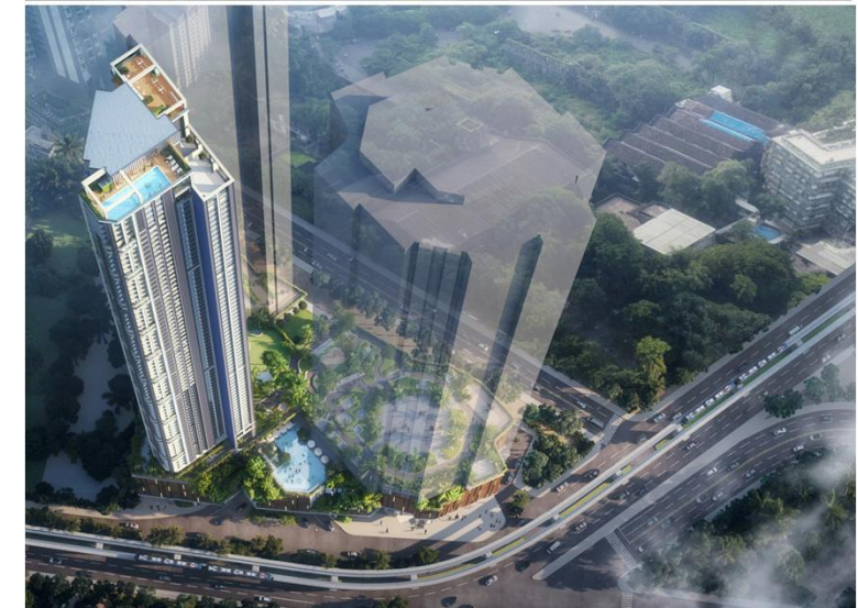
7 MAHALAKSHMI | G+82 | RUNWAL | SHREEPATI | 322 M HT STATUS: UNDER CONSTRUCTION
