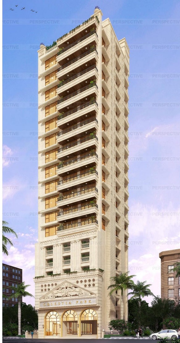
CELESTIA PARK | SHIVAJI PARK STATUS: UNDER CONSTRUCTION
