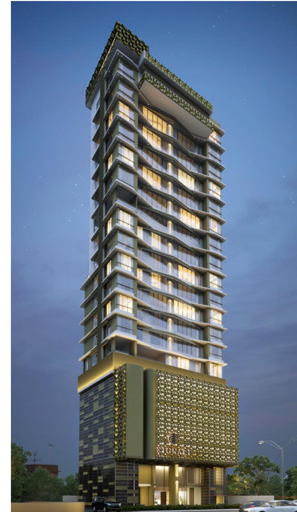
SIGNARE | DADAR | TEJUKAYA STATUS: COMPLETED
