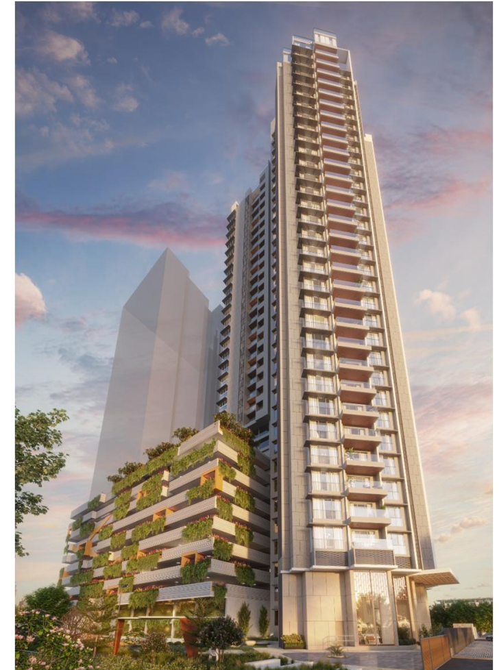
GODREJ AGARWAL NAGAR | G+34 | MATUNGA STATUS: UNDER CONSTRUCTION
